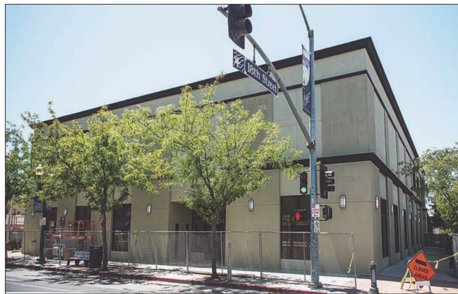
The Chester Avenue side of the newly renovated Chain Cohn Stiles building.
